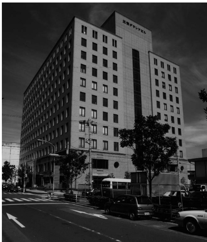
Head Office, Kobe
